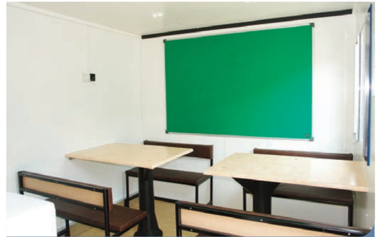
Rest area that provides comfortable bench seating for up to eight people
